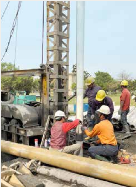
鑿井工程 Well drilling engineering
