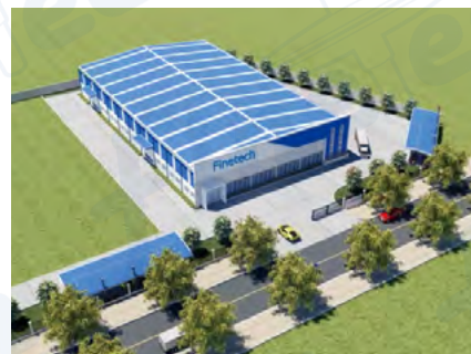
New factory under construction in Vietnam
