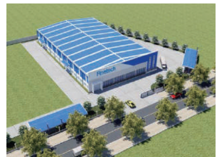
New factory under construction in Vietnam
